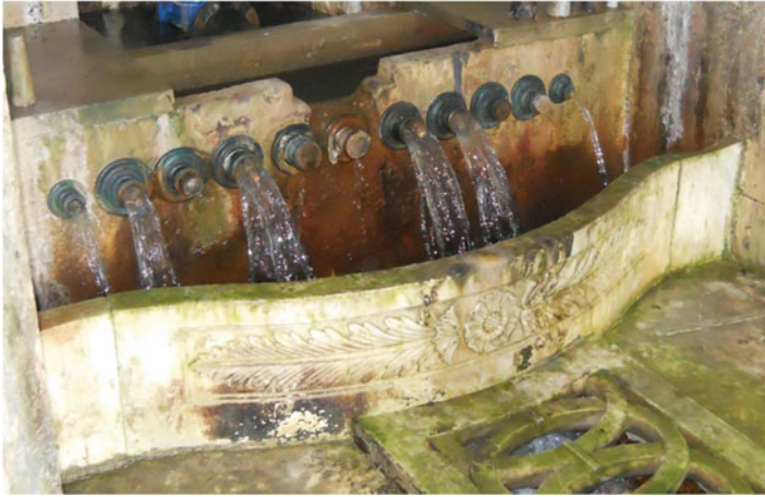
Fig. 2.26 The Orifices (lule) in the operation chamber of the Yenı Dam. (Photo by Y.Ozdemir)
